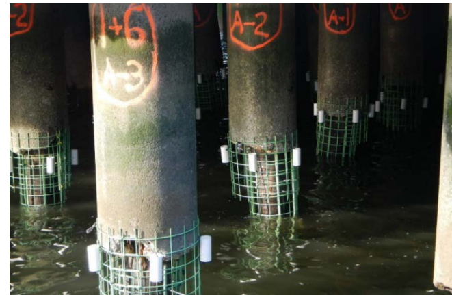
Reactive maintenance pile repair
