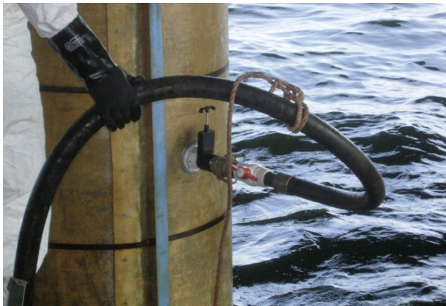
Preventative maintenance repair
